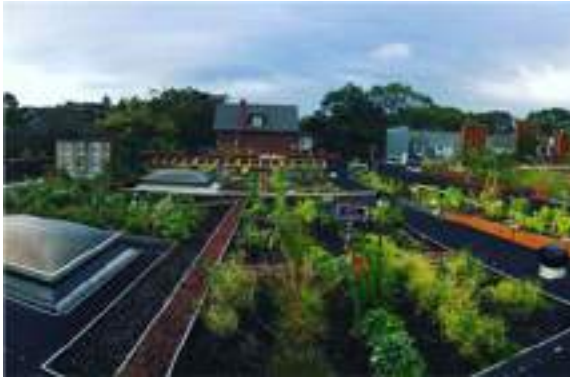
Figure 4.9 Example of a green roof (source: greenroofs.org).
