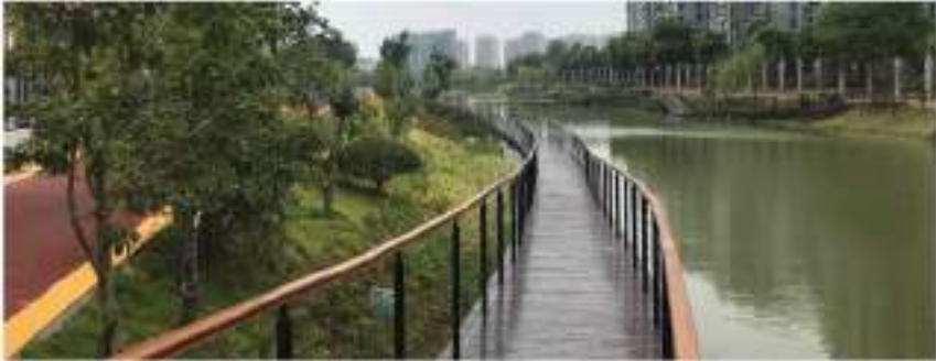
Figure 11.9 Typical view of ecological river shoreline in Chizhou City after the SCC projects (photo source: Municipal Government of Chizhou).
