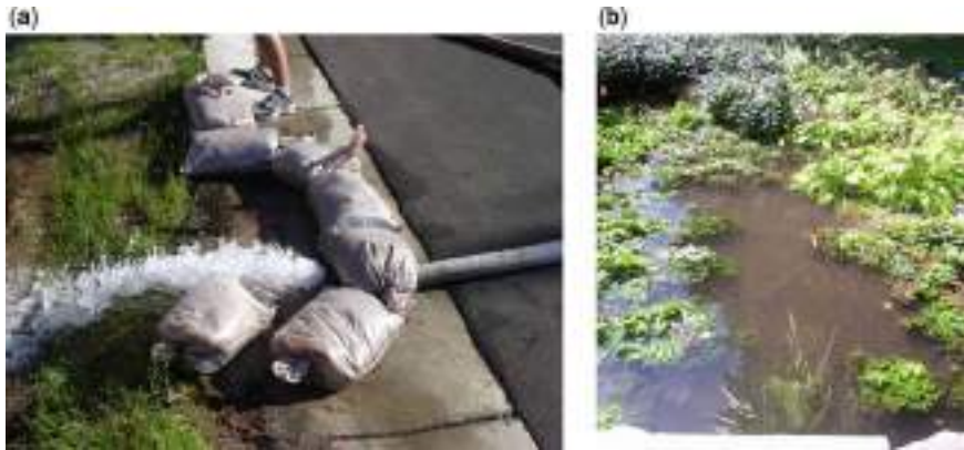
Figure 4.11 Synthetic runoff test using a fire hydrant at a rain garden. After water fills the rain garden (left), the recession of the water surface is measured over time (source: Erickson et al., 2013 ).
