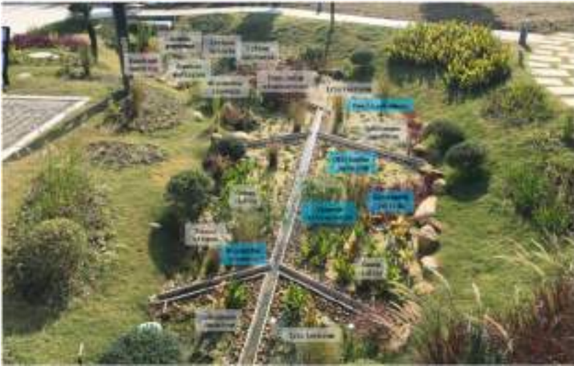
Figure 5.9 Plant distribution in the biofilter. The species highlighted in blue are ornamental species, while the rest are effective plants for pollution reduction.
