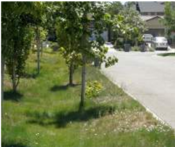
Figure 4.8 Grassed swale at the edge of a residential street without curb and gutter (source: bluegreenbldg.org).
