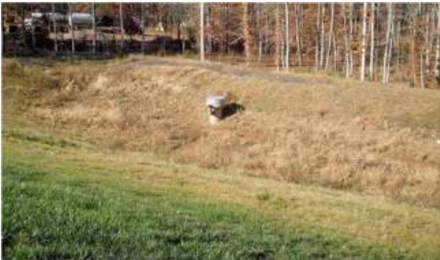
Figure 4.1 An example of an infiltration basin which can fill to the invert of the outlet structure (source: www.rivanna-stormwater.com ).
