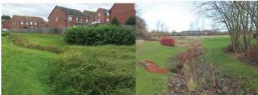
Figure 9.3 Example of a SuDS system, comprising of rock-lined swales and vegetated detention ponds, in Leicester, England. ©CraigLashford.
