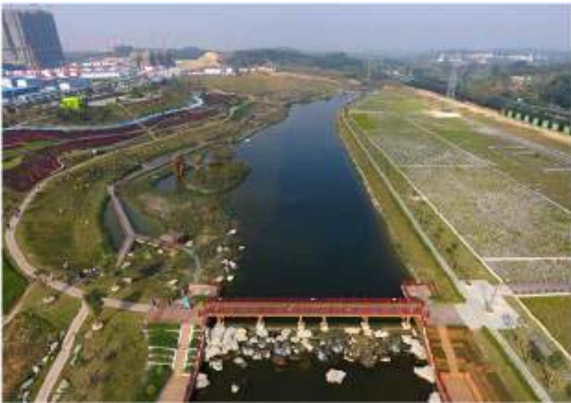
Figure 11.16 Appearance of the Nakao River after the SCC projects implementation (photo source: Municipal Government of Nanning).
