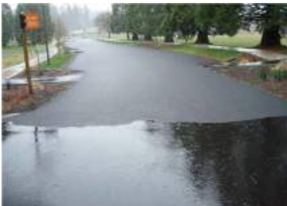
Figure 4.5 Permeable pavement (in the distance) is frequently placed on residential streets and parking lots (source: www.vaasphalt.org ).
